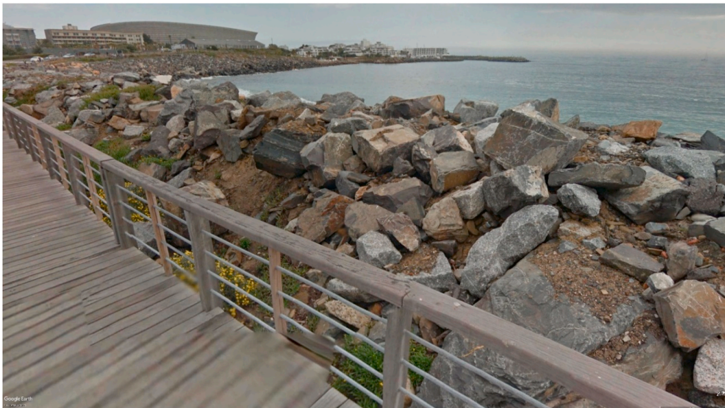
Fig. 9. Stones lined up to protect the coastline just off V&A Waterfront Source: Fieldwork (2020).
